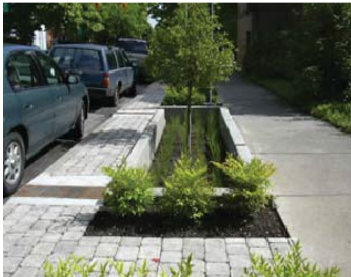
Bio-Retention in Parking Area, EPA
