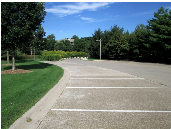
Permeable Paving, Coralville
