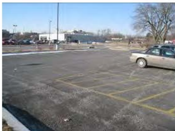
Porous Asphalt Parking (Lot 121 – Iowa State University)
