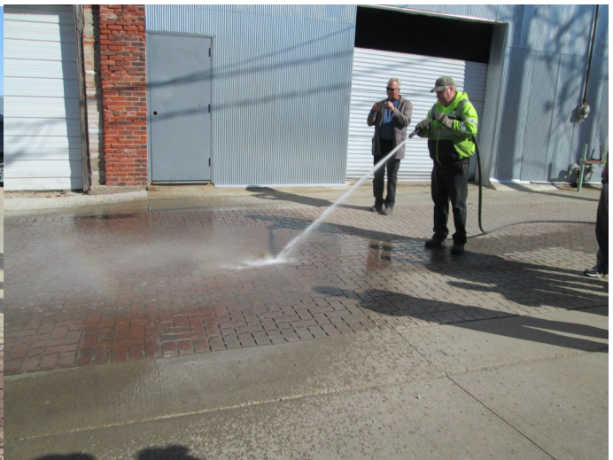
Power washing pavers to force debris out in clogged areas, Dubuque, IA
