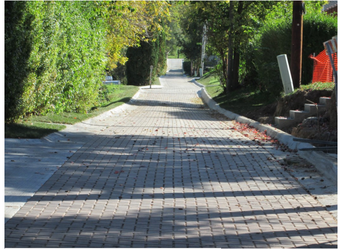
Permeable Paver Alley, Dubuque
