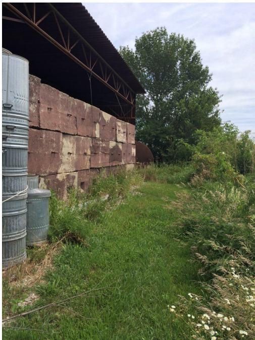
West Branch Salt Shed, South Wall
