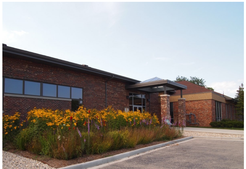
Example of rain garden at Town Hall in Somers, Wisconsin
